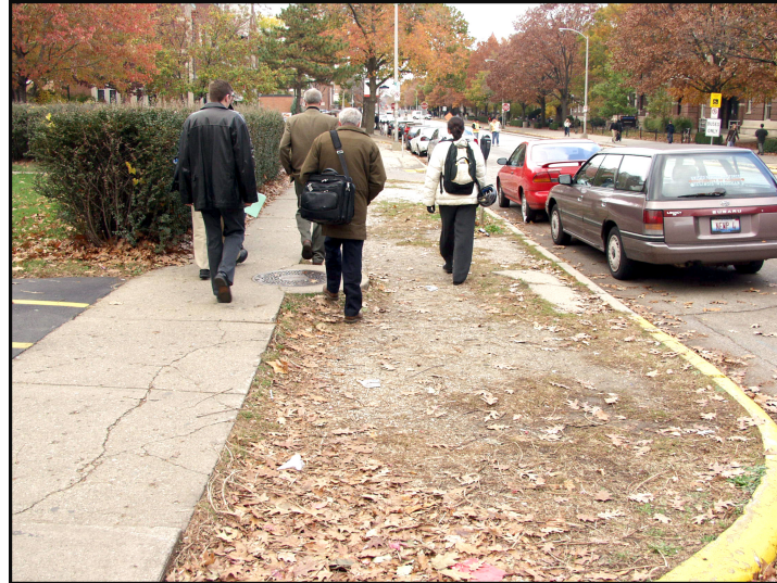
Insufficient sidewalk widths for high pedestrian traffic areas.
